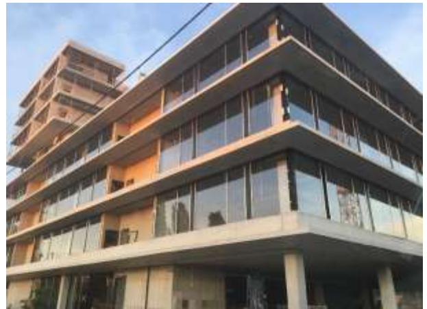
Figure 4: Alpha Centauri (Infobip) under construction
