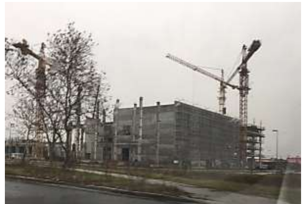
Figure 5: Buzin City Island under construction
